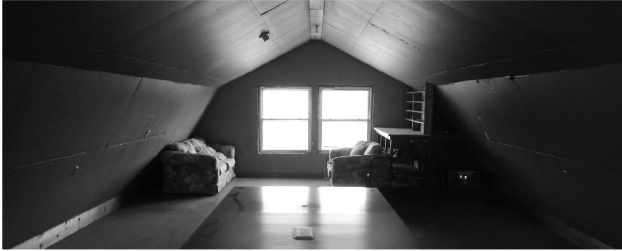
1 BUILDING #9 (BARN) - EXISTING UPPER FLOOR - INTERIOR VIEW SCALE: NOT TO SCALE
